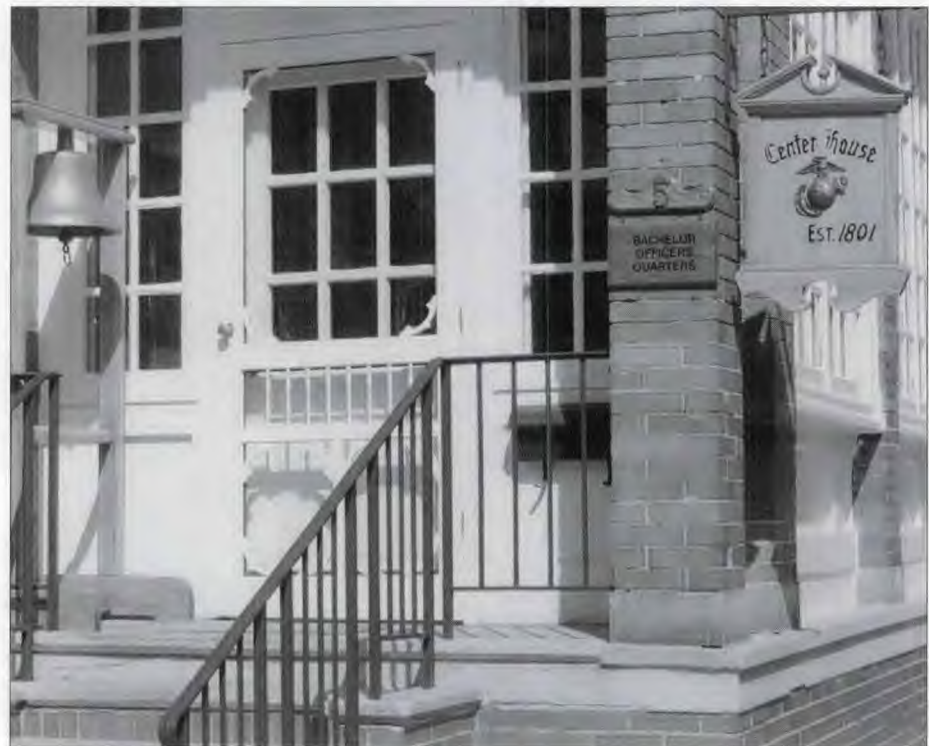
Historic Center House links barracks officers past and present. (photo by Pfc. Elizabeth A. Thomas)
