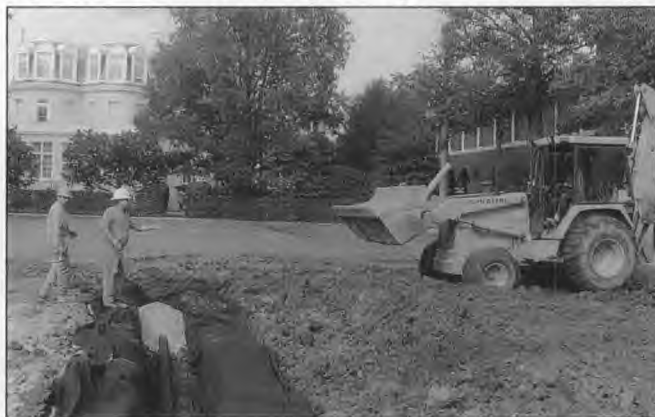
Construction workers cover the newly installed drainage system before laying sod. (Photo by LCpl. Matt Schafer)
