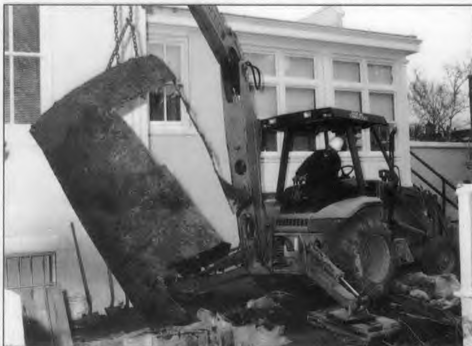
A worker uses a backhoe to remove one of two fuel oil tanks from next to the Home of the Commandants. The tanks had been in place for at least 40 years, and were no longer needed when a gas heater was installed in the house. (Photo by LCpl. Joey D. Benford)
